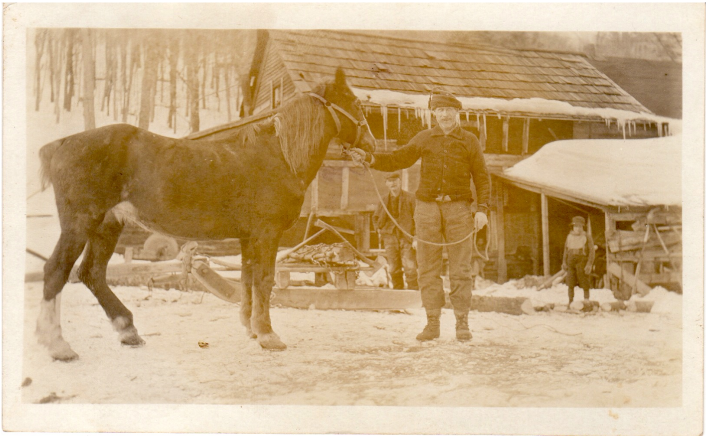
Can you identify this photo?? It appears to be a logging camp but we don't know where it is and who the people are. The photographer is George W. Gale.
